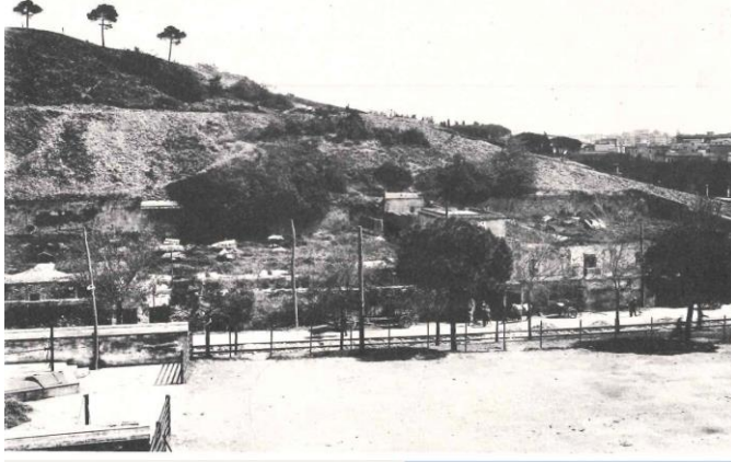
Fig. 8: Monte Testaccio – cross-section of the waste heap in one sector. AUT Archivio Urbano Testaccio in Rodriguez Almeida 1984)
