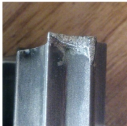
Fig.6. Repaired area before machining.
