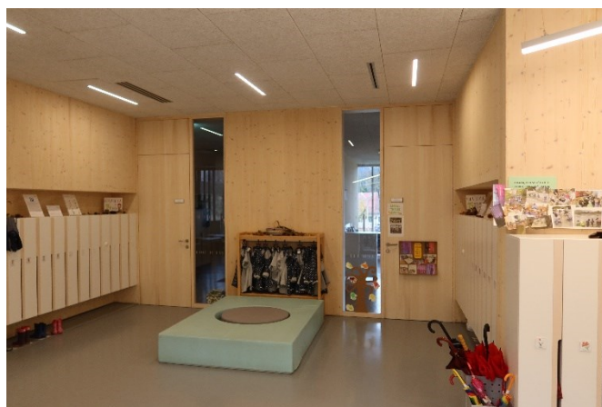
Fig. 12. Hallway space and a view of the playroom with CLT load-bearing panels with a fine finish. (Photo: Jakub Hanták, 2021)
