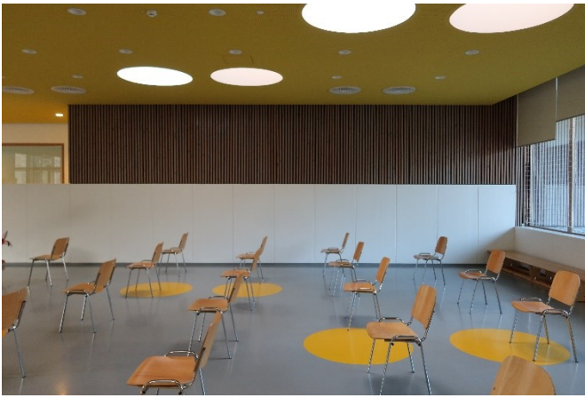
Fig. 6. Wooden perforated cladding, improving the acoustic conditions in the entrance hall. (Photo: Jakub Hanták, 2021)
