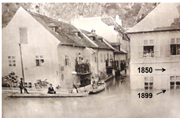
Fig. 6. Zuckermanel – Ballusova St. in 1899 – flood mark of the February 5 th , 1850 flood, and water level of the 1899 flood (photo: adopted from the City Gallery of Bratislava).
