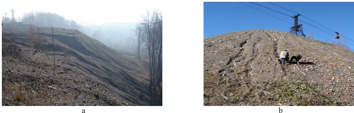
Figure 2. Lupeni (a) and New Uricani Funicular (b) dumps affected by erosion, landslides and uneven settlement [9].
