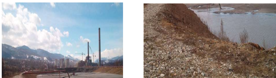
Figure 3. The settling pond of the Paroșeni thermal power plant [5]
