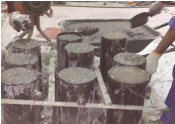
Fig. 2. Concrete cylinders during casting
